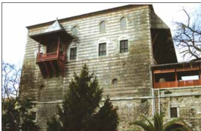
Figure 9: The façade of the Palace of Ibrahim Pasha's Divanhane and view of the balcony.
