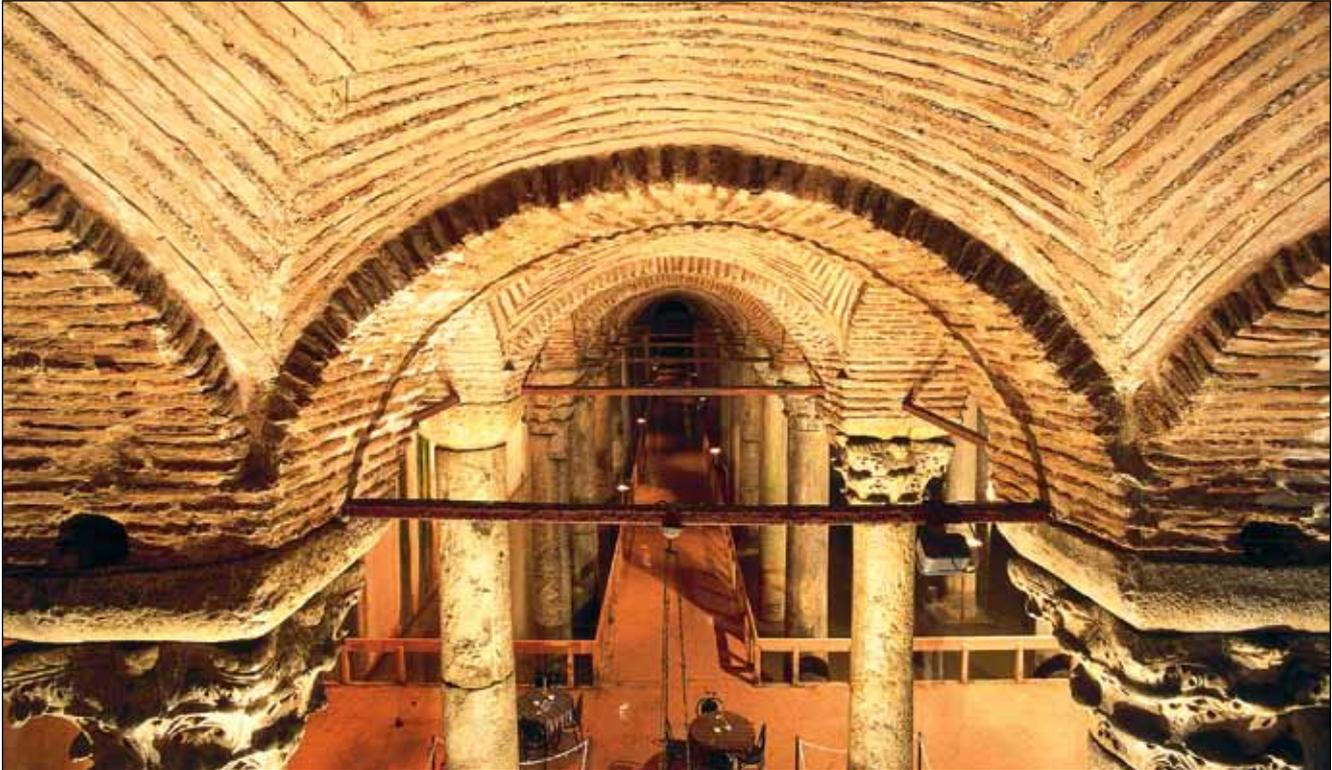
**Figure 1:** View from the platform and arches at Yerebatan Palace that were built after the restoration works and allow visitors to tour without damaging the structure.
